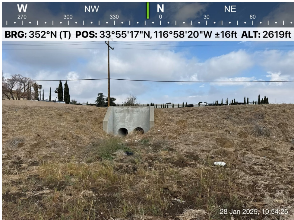
Photograph 14: Culvert passing under 1 st Street on south side where empties into low lying field.
