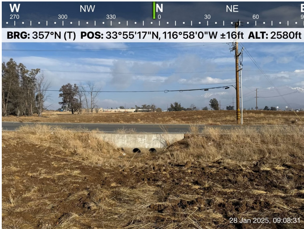
Photograph 2: Culvert on south side of 1 st Street.
