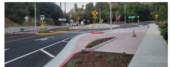
Avenue 64 Complete Street in Pasadena, CA.
