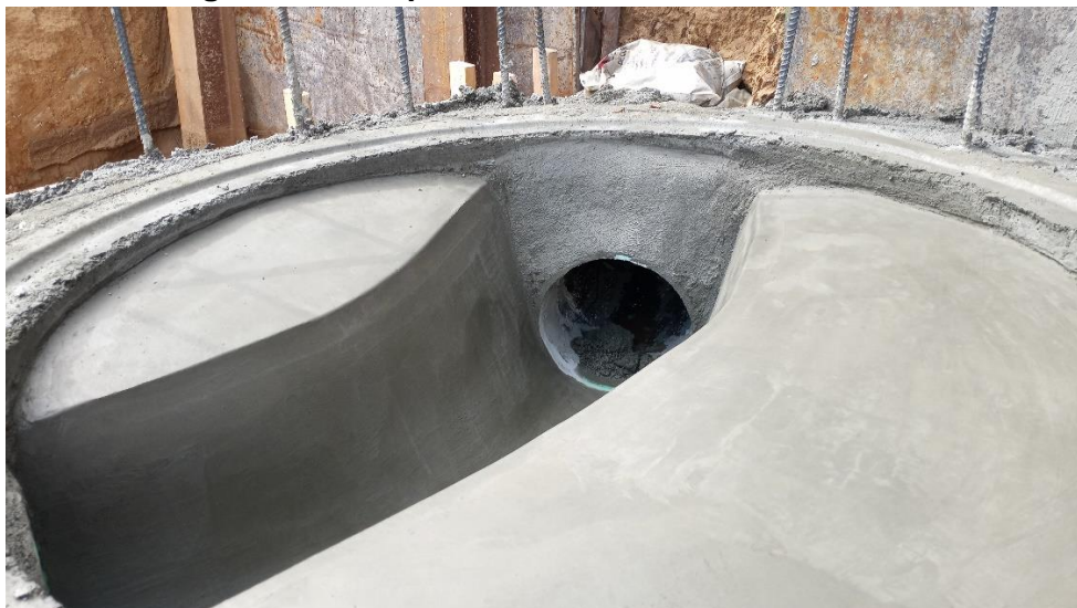
Figure 2 - Manhole bottom with full-height channels
