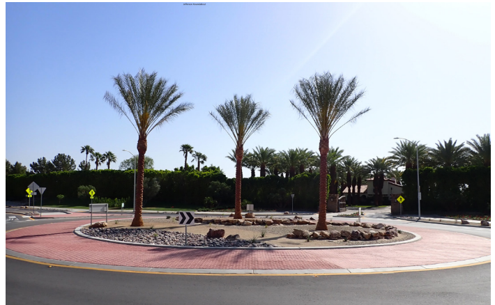
Jefferson Street/Avenue 53 Roundabout
