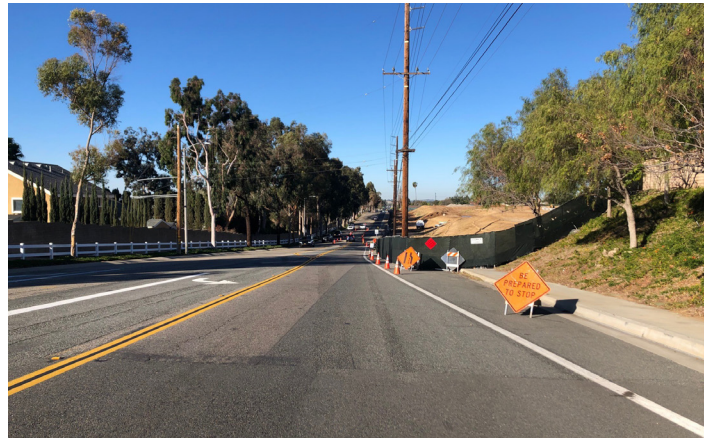
Bastanchury Road Widening
