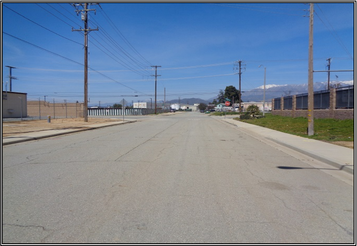
View north along Elm Avenue
