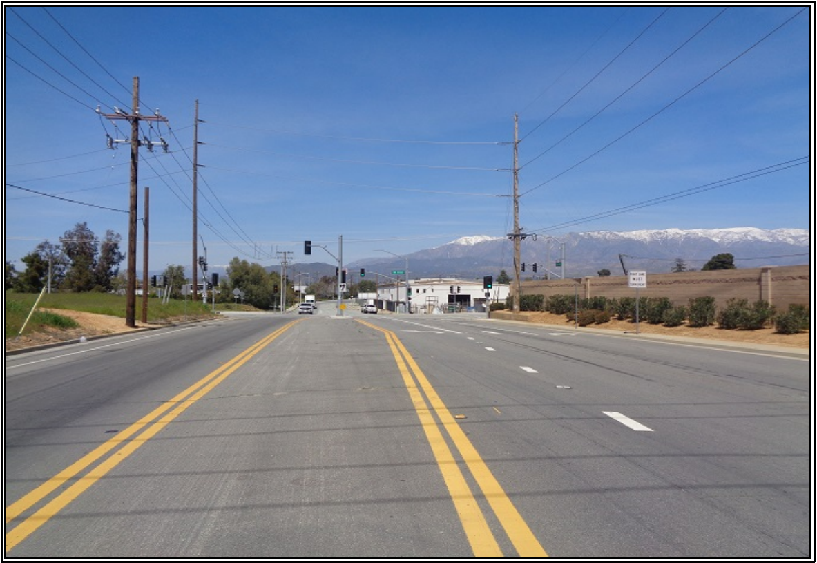
View north along Viele Avenue
