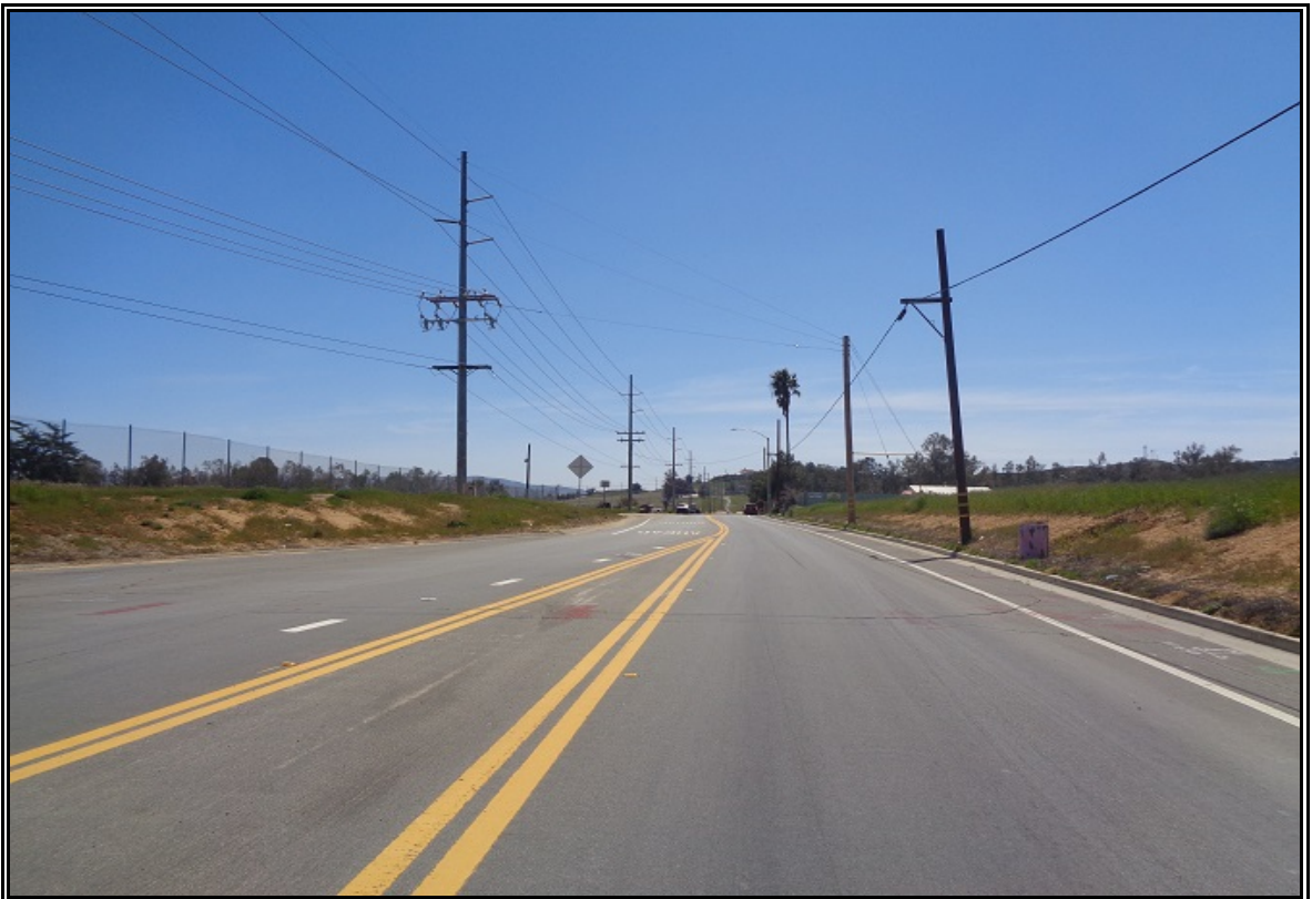
View south along Viele Avenue
