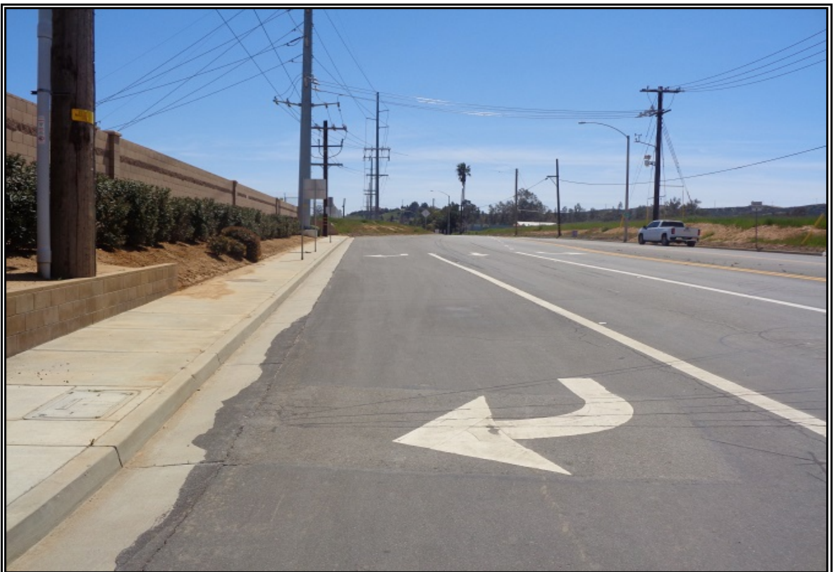
View south along acquisition area
