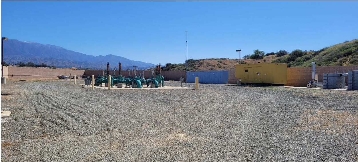
Photograph No. 1: Present site conditions, facing southeast
