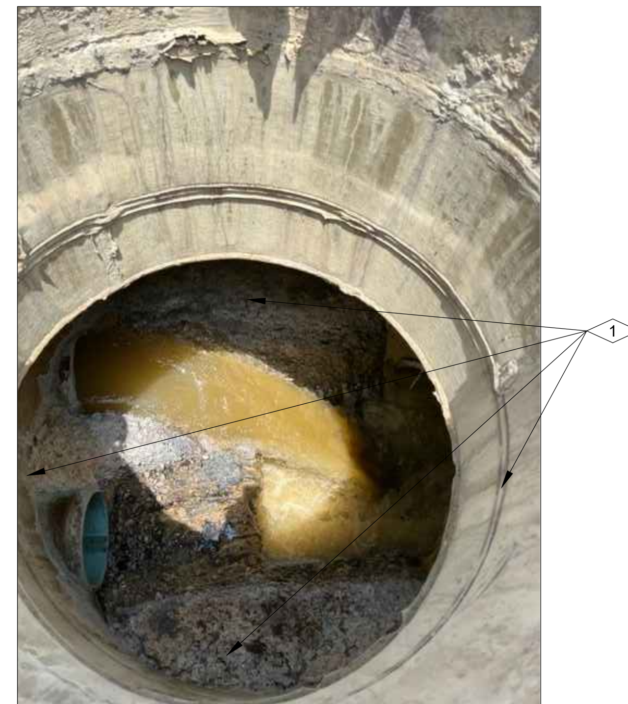
MANHOLE #4 INTERIOR PHOTO NTS
