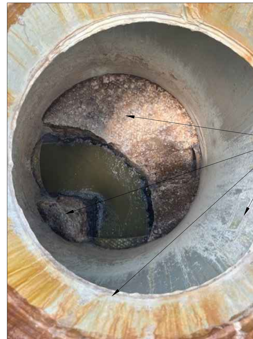
MANHOLE #2 INTERIOR PHOTO NTS
