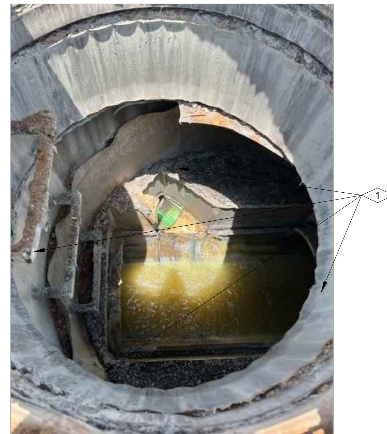
MANHOLE #3 INTERIOR PHOTO NTS
