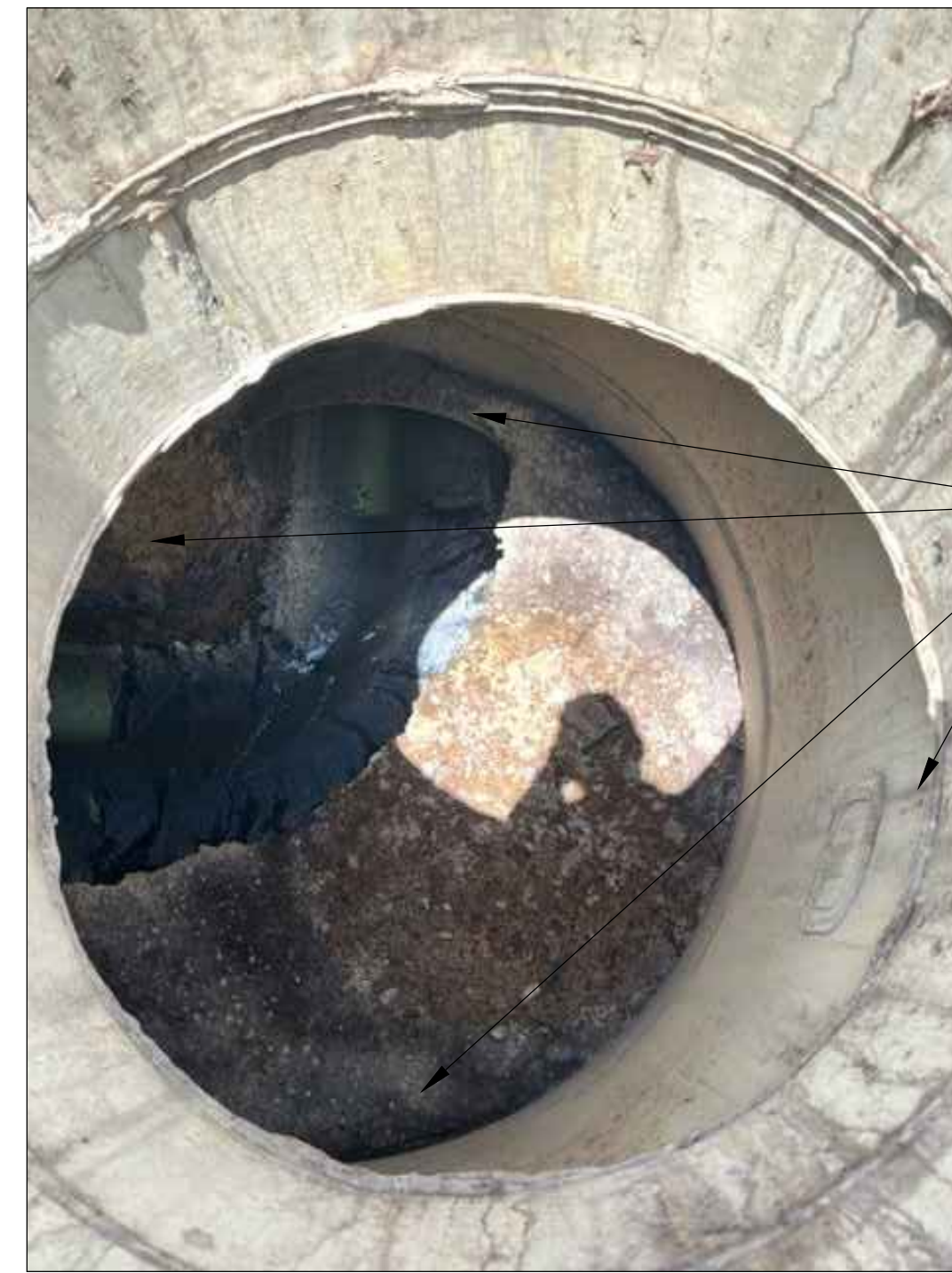
MANHOLE #1 INTERIOR PHOTO NTS
