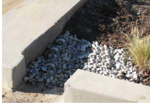
Figure 2: Curb Cut located in a Bioretention Facility
