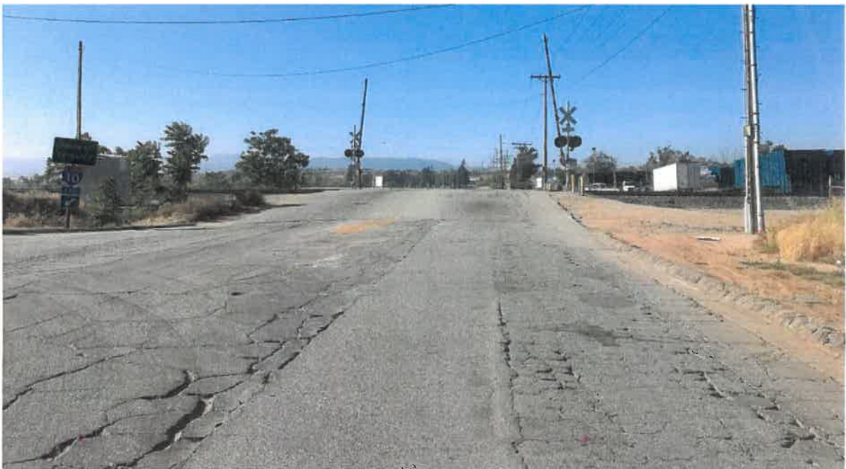
Photo No. 4: This photo shows the train crossing zone facing south.
