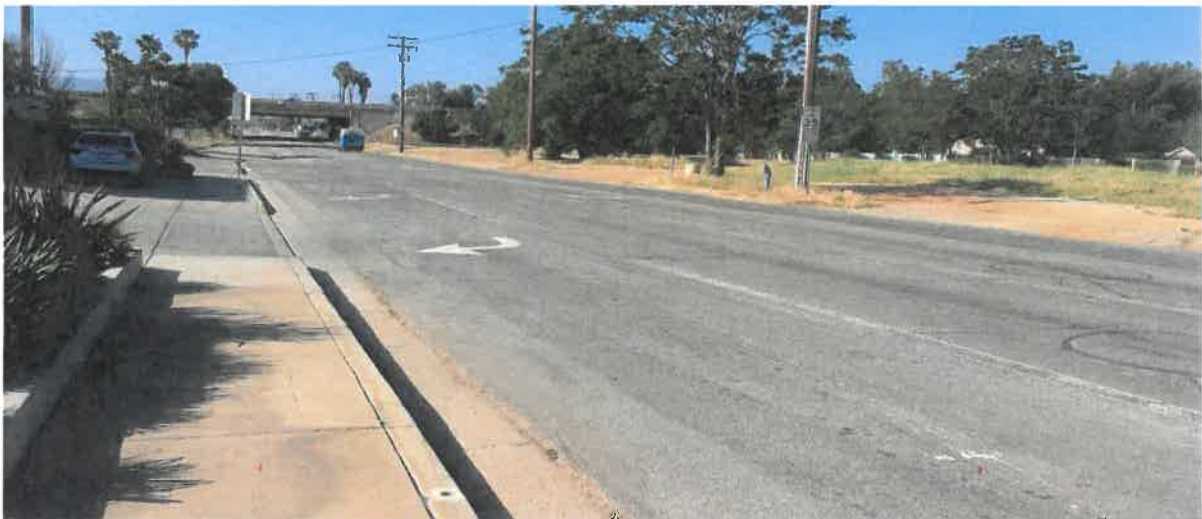
Photo No. 2: This photo shows the conditions on Pennsylvania Ave. from 6 th St. facing southwest.
