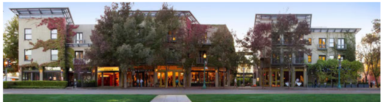
An example of a single mixed use project with varied massing connected by a datum of shade canopies, awnings, trellises, and storefront lintels (top edges). This complex is approximately the width of a 6th street block frontage. This example uniquely represents a national folk architecture with elements of early 20th century modern.
