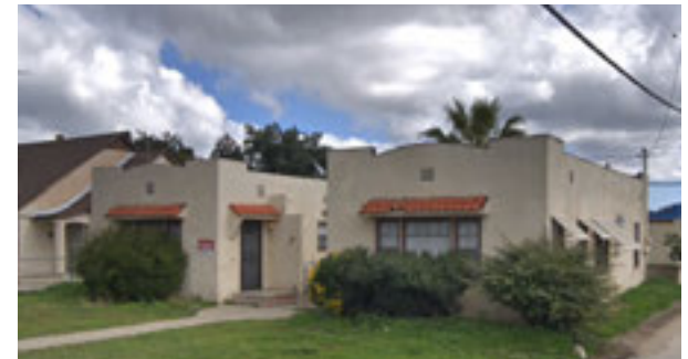
Historic downtown bungalow court housing, Beaumont, CA
