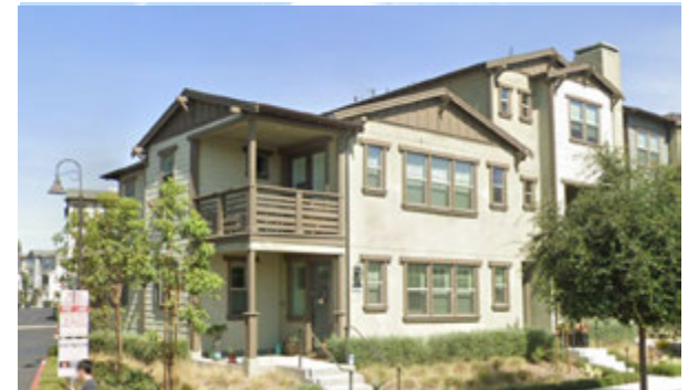
3-level multifamily (townhomes), Tustin, CA
