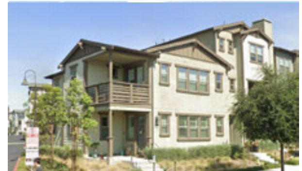
3-level multifamily (townhomes), Tustin, CA
