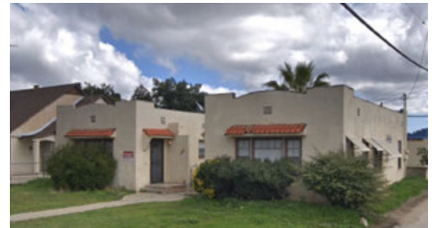
Historic downtown bungalow court housing, Beaumont, CA
