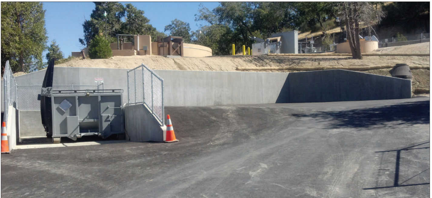
Photo 7 - WEBB designed Lake Arrowhead Community Services District's Vector Truck Dump station for the Willow Creek Wastewater Treatment Plant
