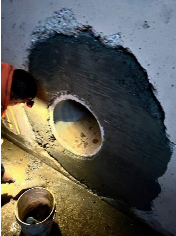
Interior Storm Structure-1
