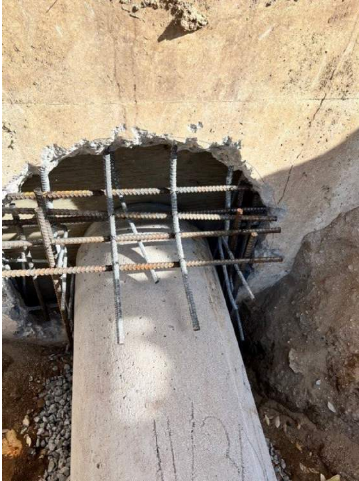
Rebar Installed-3
