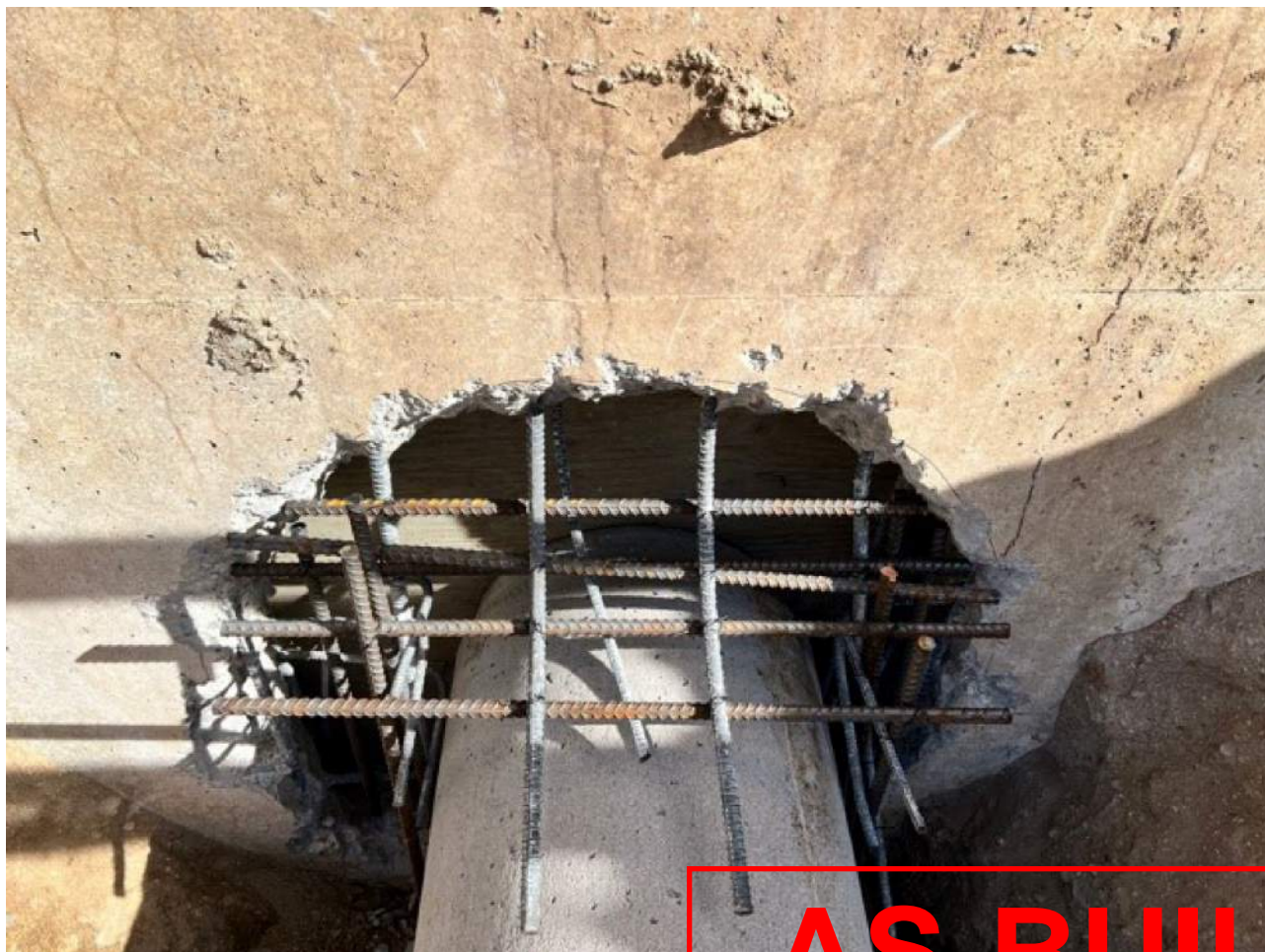
Rebar Installed-2
