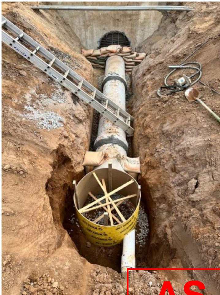
Manhole to Storm Structure 2 of 5
