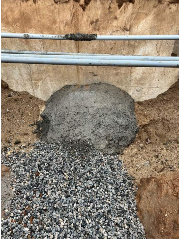
Exterior Storm Structure
