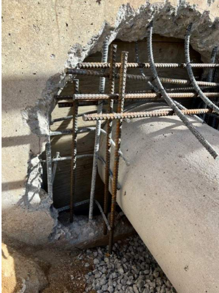
Rebar Installed-5
