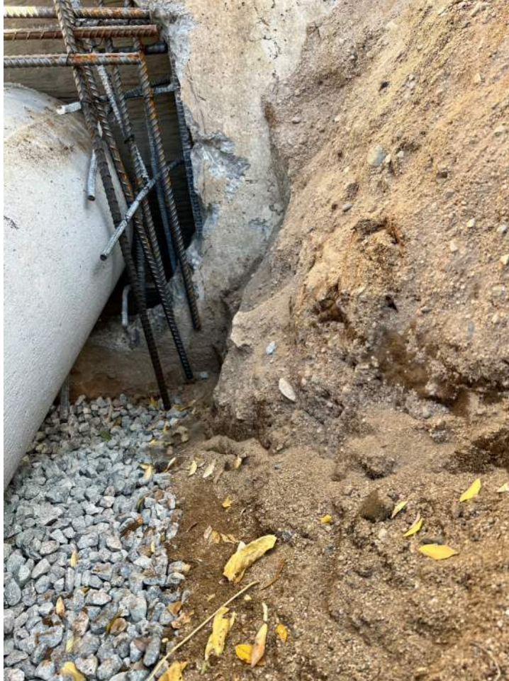
Rebar Installed-1
