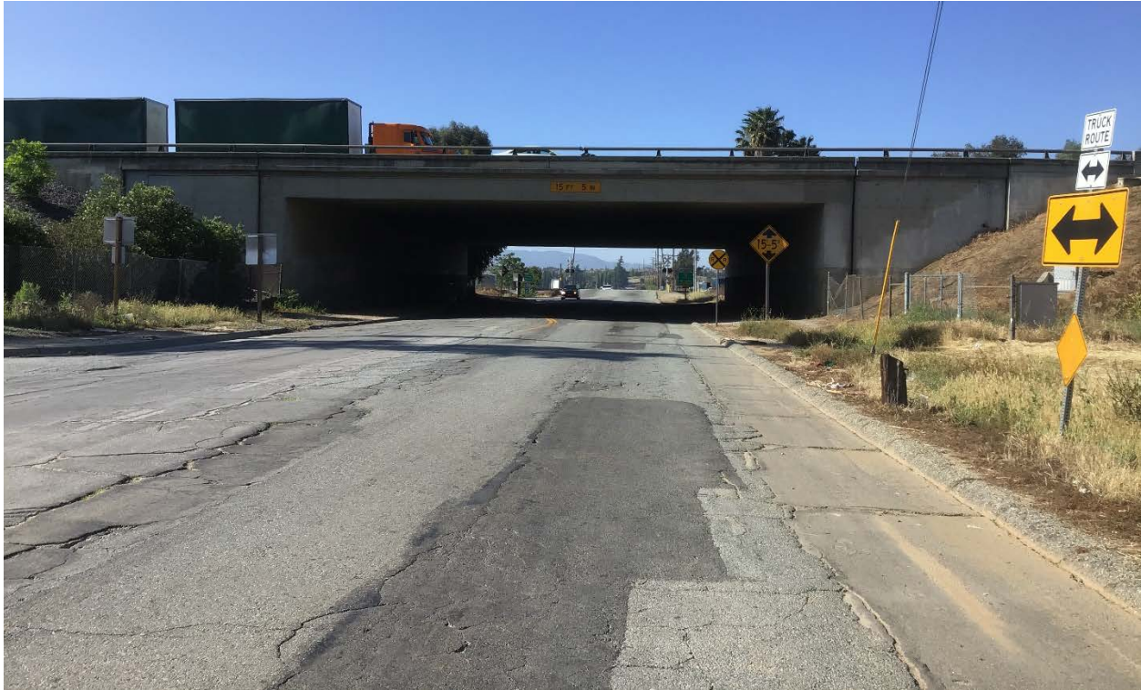
Photo No. 3: This photo shows the freeway overpass facing south.
