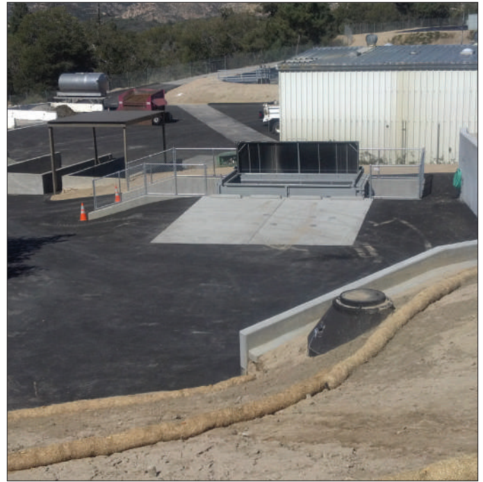
Photo 6 - Willow Creek Vector Station, Lake Arrowhead Community Services District - Showing a roll-off dumpster with an integrated screen to remove solids from the liquid prior to discharging the liquid into the influent sewer.
