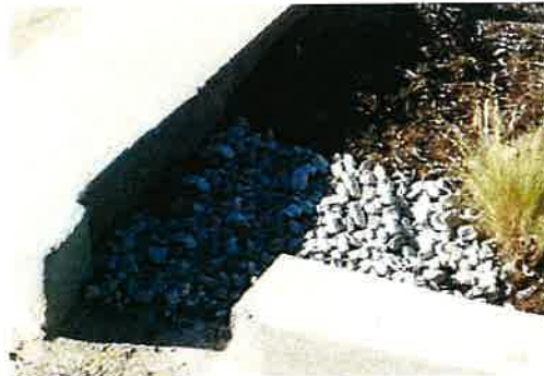
Figure 2: Curb Cut located in a Bioretention Facility
