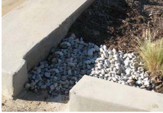
Figure 2: Curb Cut located in a Bioretention Facility
