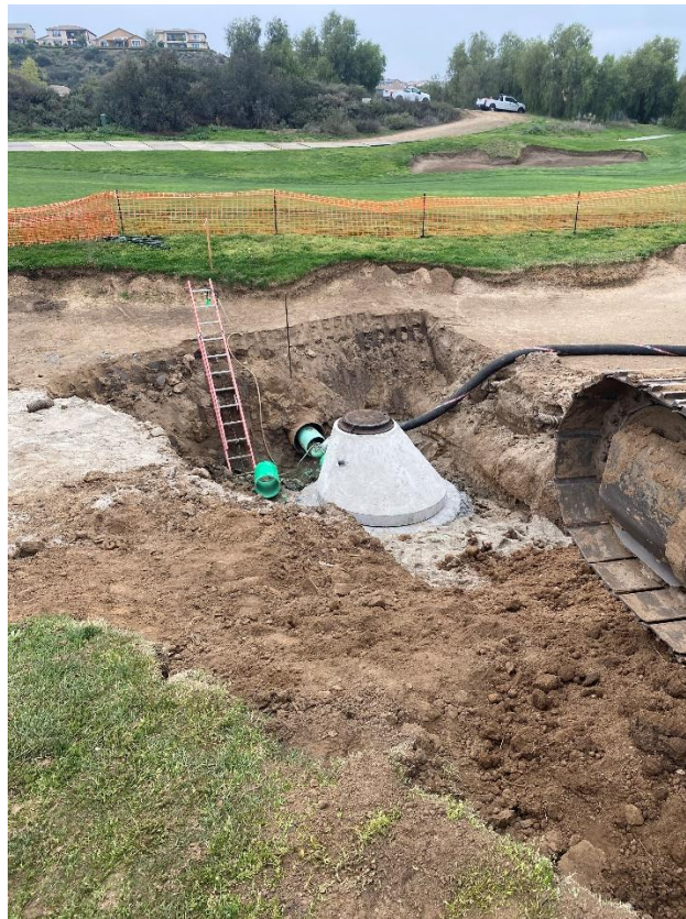
Figure 1 - Completed manhole cover located by the sand trap
