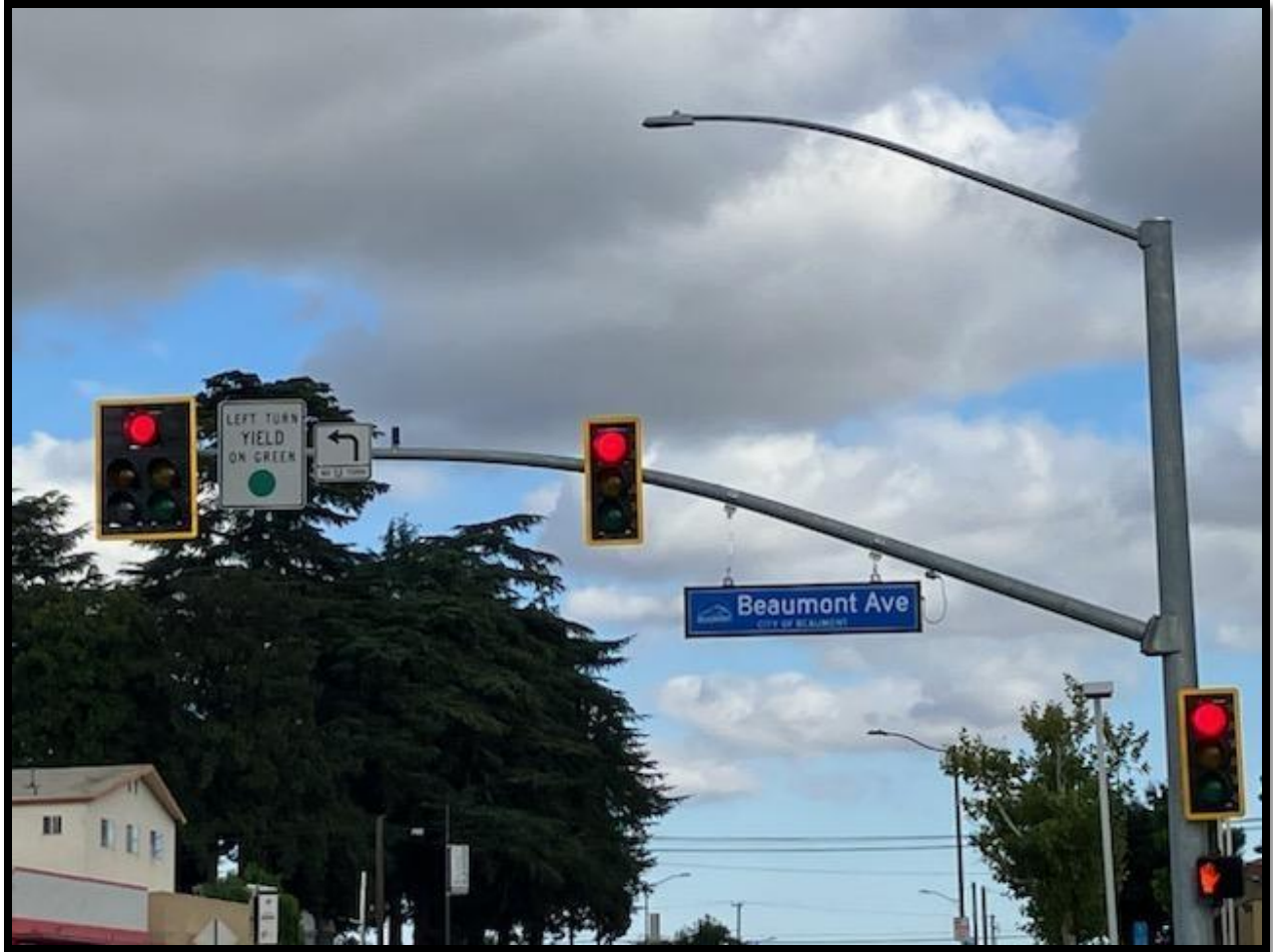
Figure 1 - Beaumont Avenue and Sixth Street Traffic Signal
